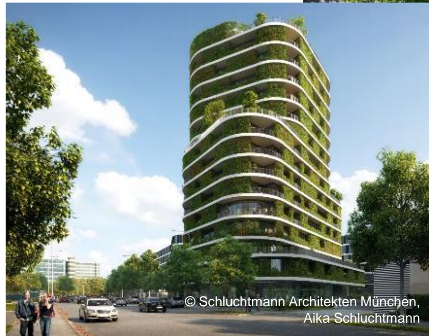
Arabella Hochhaus in Munich (being built)
