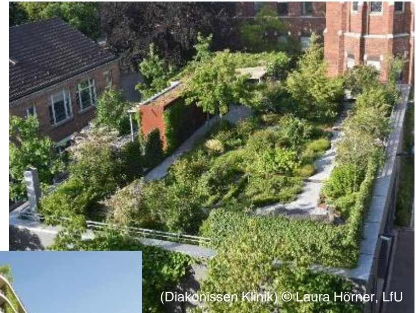
Intensively-used Green Roof in Augsburg
