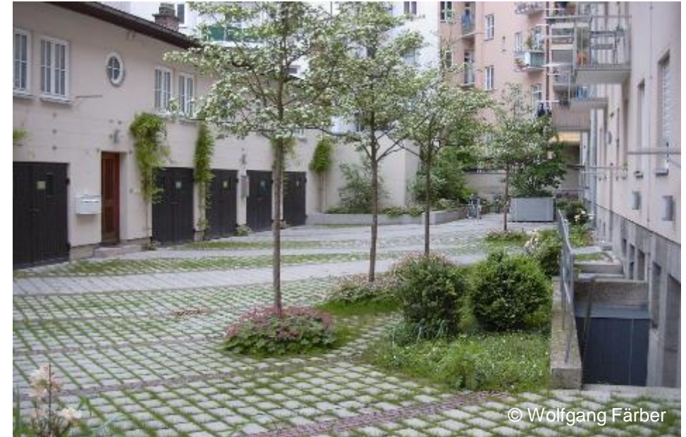
Water-permeable parking spaces
